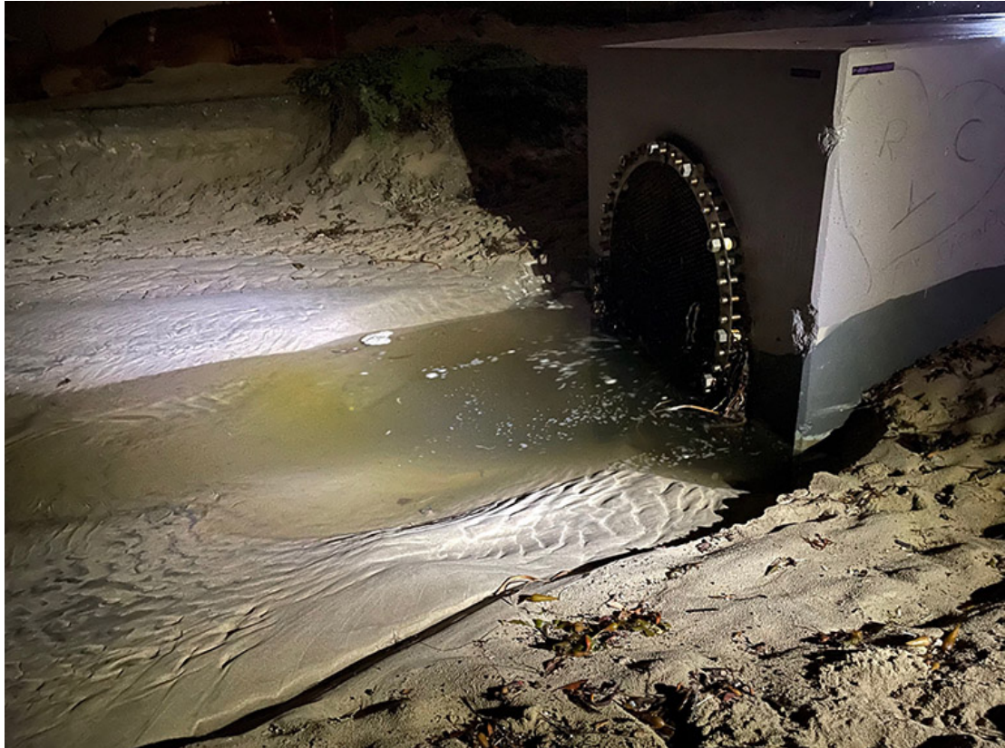
Figure 3. Bay Street (Seaside and Sand City) during the First Flush on December 17 th , just as the end of the pipe further down the beach becomes unblocked and water is sucked back through the “tower”. When the end of the pipe is blocked by sand, water comes out the “tower” and flows down the beach to clear the end of the pipe: a duck-billed flange at the end of a 90” pipe. Photo: Lisa Emanuelson.
