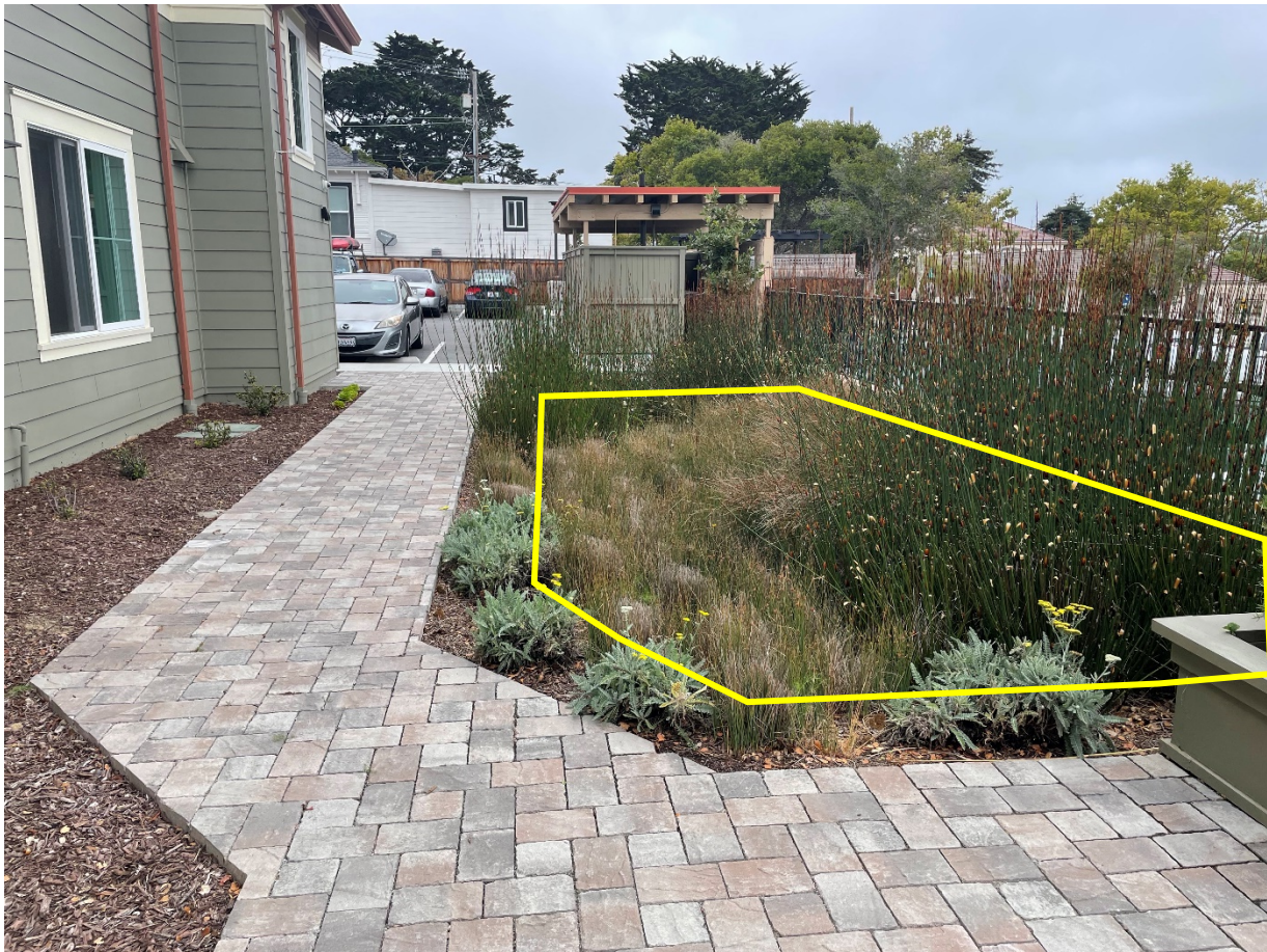
A 6"-deep bioretention planter
