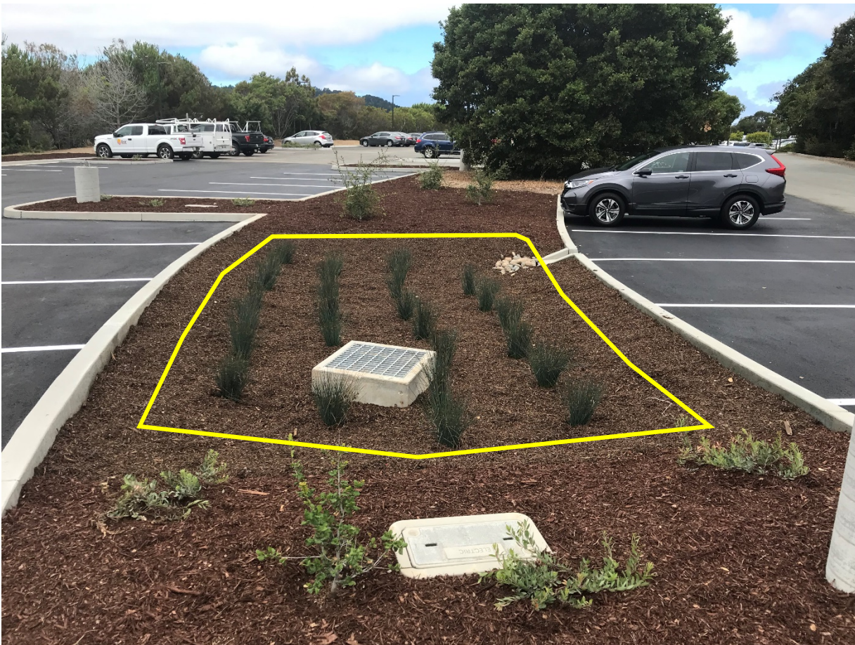
A 6"-deep bioretention planter
