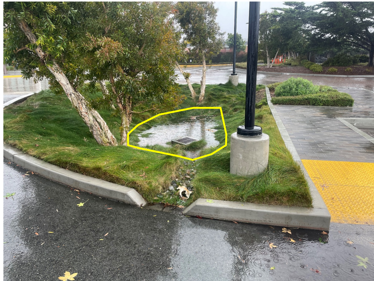
A 2'-deep bioretention planter (still only ponds 6" deep)
