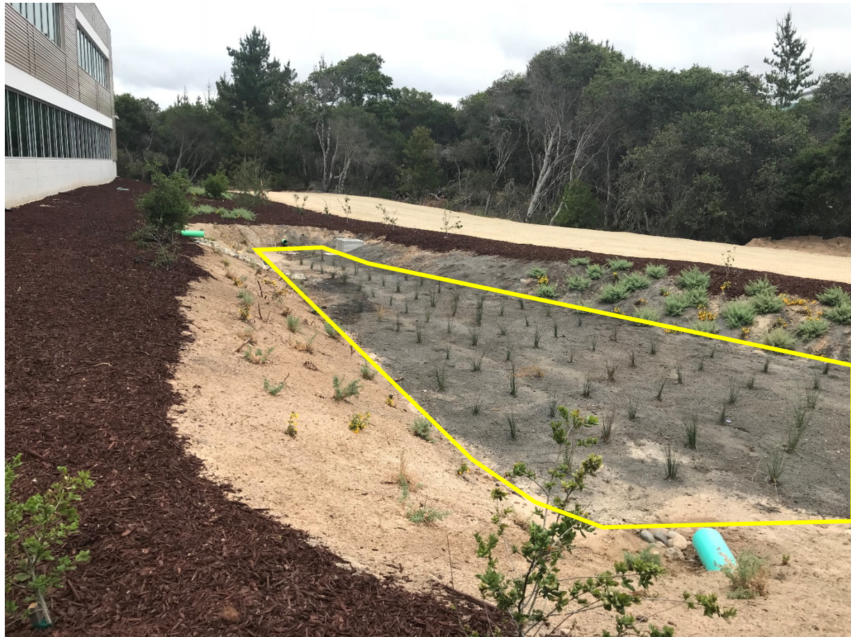
A 2' to 3'-deep bioretention planter (elevation varies around perimeter)
