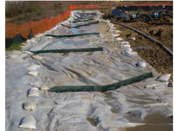
Plastic check dams are used to reduce runoff velocity and to control erosion and sediment displacement.
