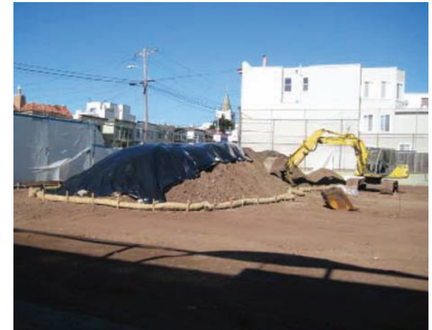
Fiber rolls are properly installed around a stockpile.
