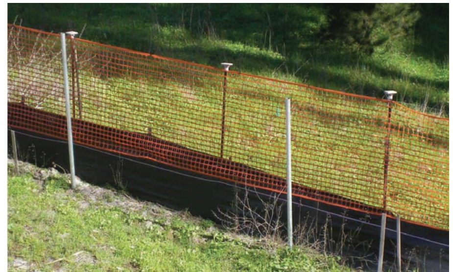
Silt fence is properly installed along the slope to intercept sheet flow.
