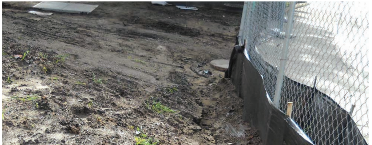
Silt fence is attached to construction fencing to prevent sediment from leaving the site.
