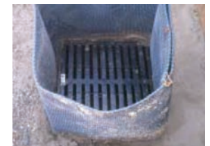
Properly protected inlets
