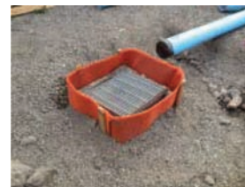
Properly protected inlets
