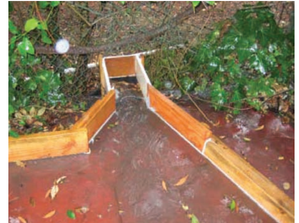
A temporary diversion structure was built upstream from a steep slope. It prevents runoff from flowing down the slope and causing hillside erosion.
