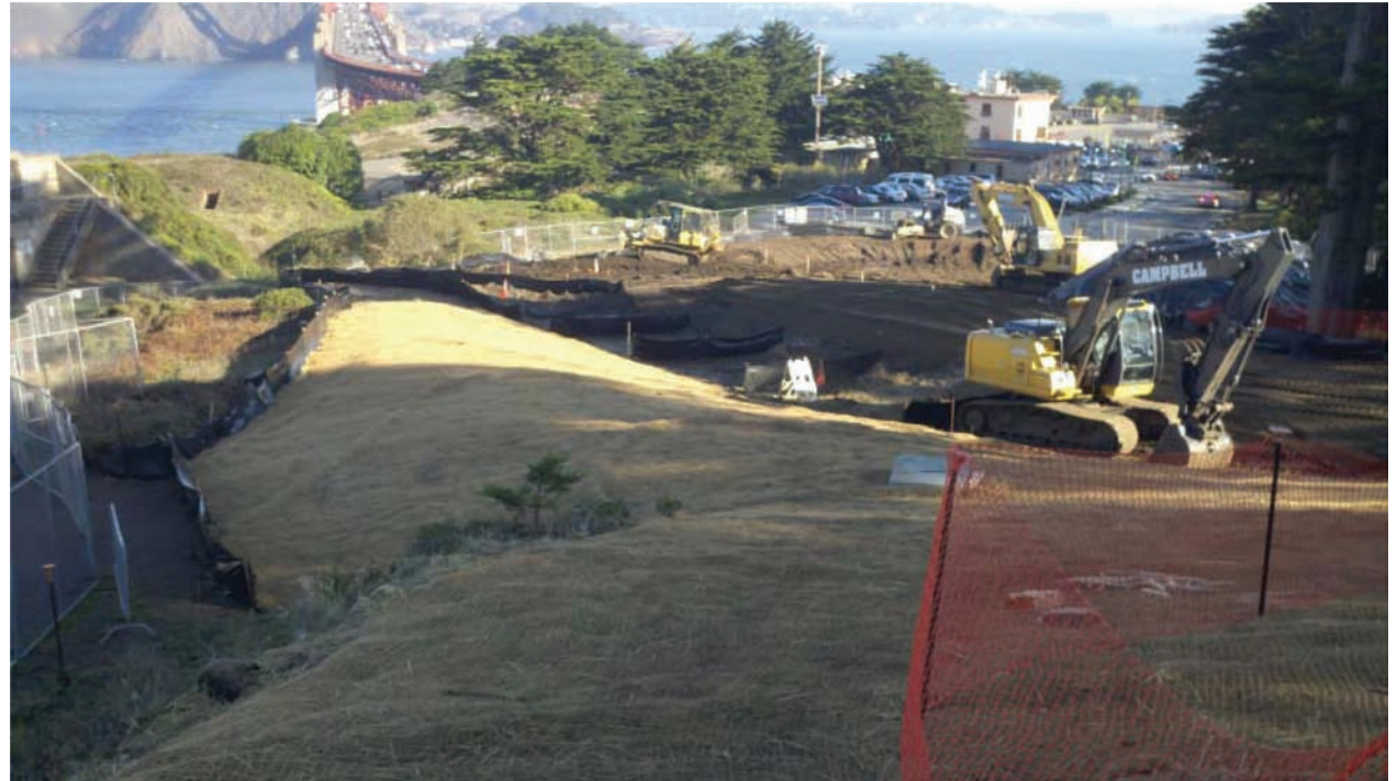
Jute netting was placed along these slopes to prevent erosion prior to the establishment of vegetation.
