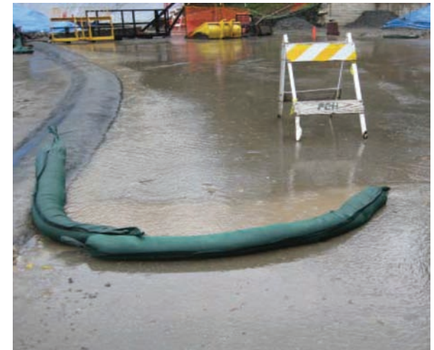
Gravel bags are used to form a check dam along the roadway.
