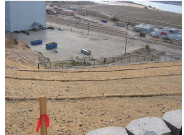
Hydroseed was applied to the hillside to provide stabilization.
