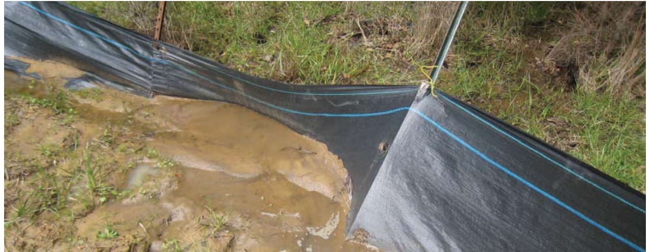
This silt fence is not properly installed and sized causing failure.
