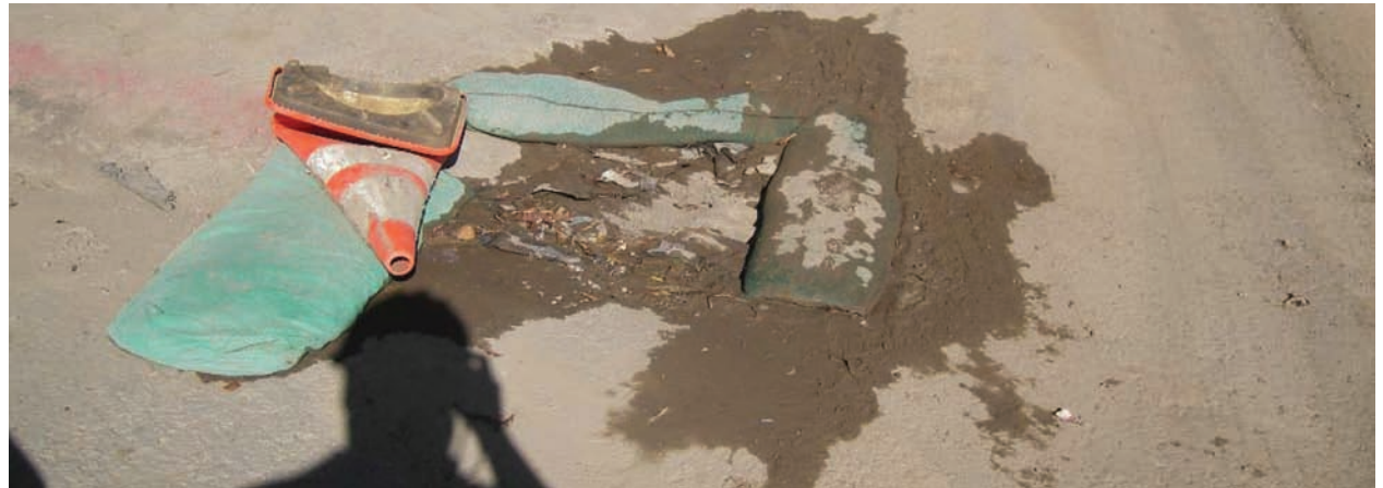
Inspect and maintain all BMP's to ensure that they perform well, and do not fail like this gravel bag berm.
