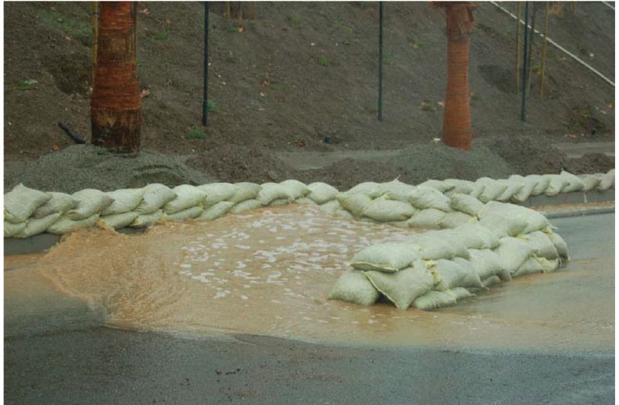
A gravel berm is being used to slow the runoff and filter out sediment.
