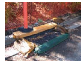
Properly protected inlets
