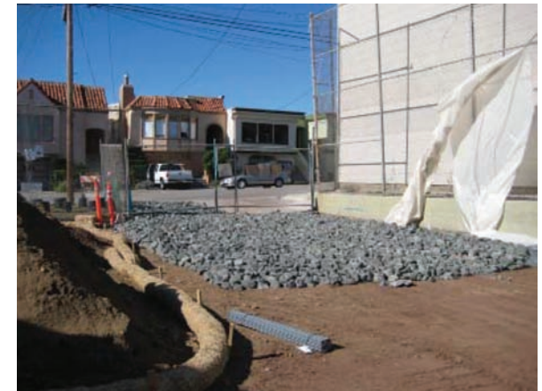
A gravel construction access is properly installed at the site entrance.
