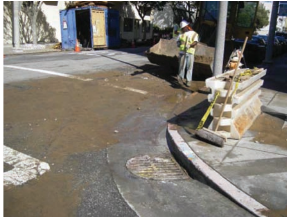
Site violations: unprotected inlet, tracking mud and concrete waste.
