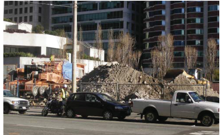
Water is applied to exposed soil and stockpiles to prevent dust generation.
