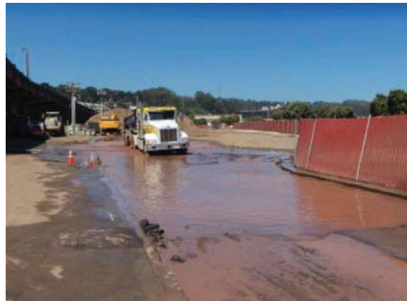
Construction area without a tire wash.
