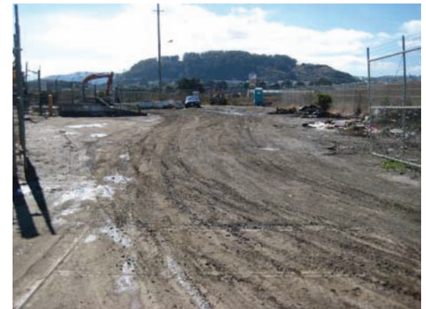
The entrance to this site requires a stabilized roadway.
