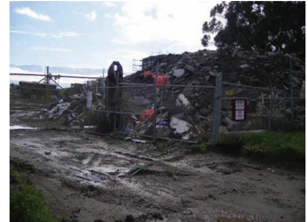
The entrance to this construction site is unstabilized, and will promote dirt tracking.
