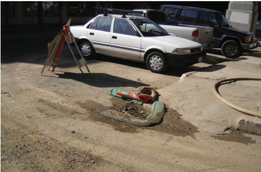
The BMP at this drain inlet needs replacement and ongoing maintenance. Sediment, debris and other pollutants can easily enter the storm drain system.
