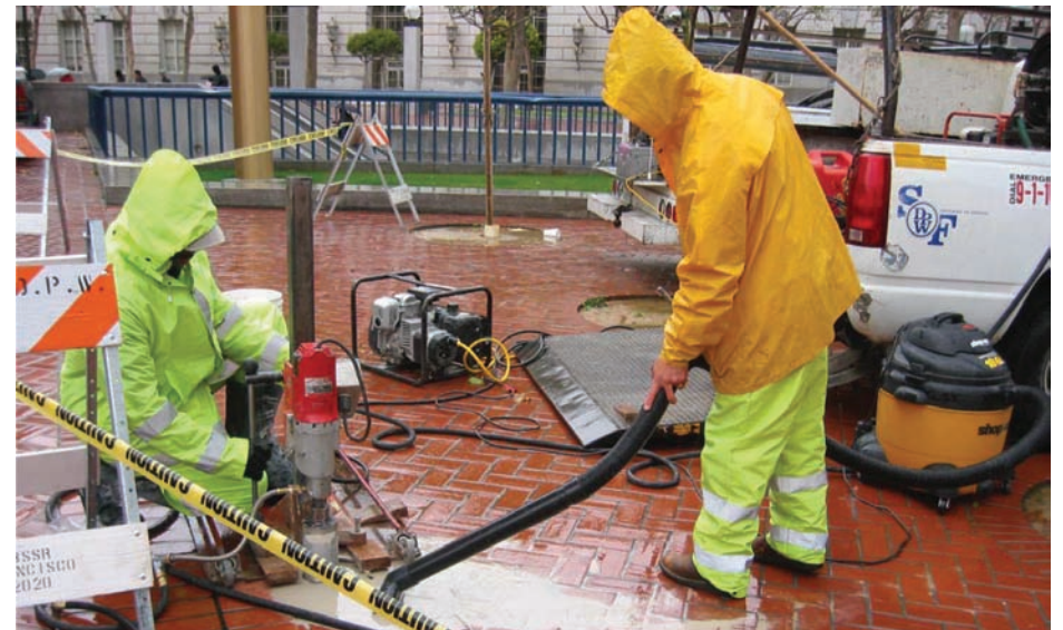
Workers vacuum liquid waste from drilling activities.
