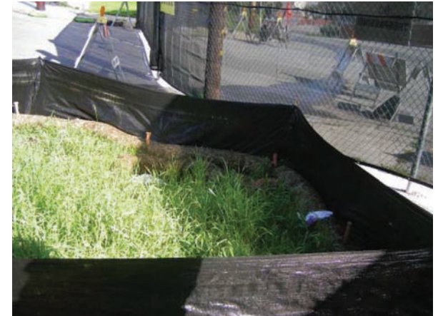
Existing vegetation is protected with fiber rolls and silt fence.
