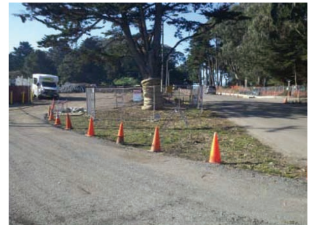
An existing tree is protected with fiber rolls and perimeter fencing.
