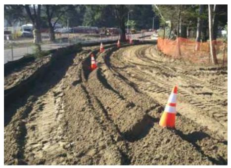
Soil roughening was used on this construction area to prepare for vegetative establishment.
