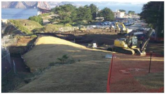
Jute netting was placed along these slopes to prevent erosion prior to the establishment of vegetation.
