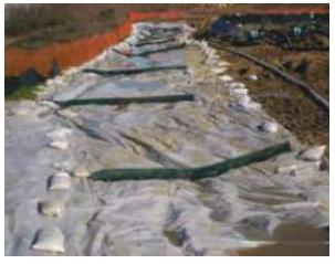
Plastic check dams are used to reduce runoff velocity and to control erosion and sediment displacement.
