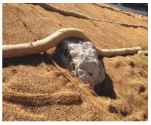
Remove or by pass all obstructions prior to placing fiber roll. Do not install the roll over the obstruction.
