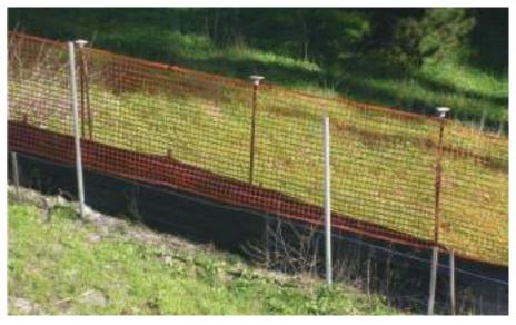
Silt fence is properly installed along the slope to intercept sheet flow.
