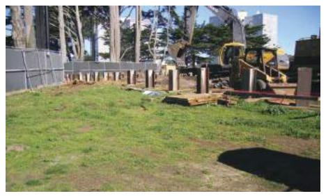
Extend the silt fence to the top of the perimeter fencing. This provides wind control and site security.
