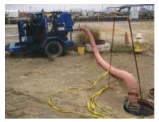
Contractors are illegally pumping unfiltered site runoff directly into the storm system.
