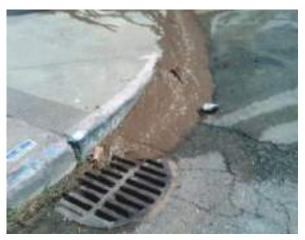
Untreated runoff from an upstream construction site is being discharged to the City storm system.
