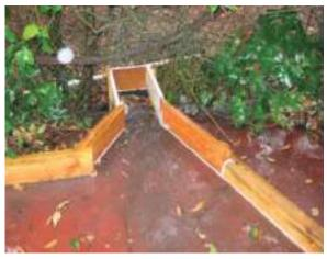
A temporary diversion structure was built upstream from a steep slope. It prevents runoff from flowing down the slope and causing hillside erosion.
