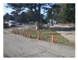
An existing tree is protected with fiber rolls and perimeter fencing.
