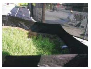
Existing vegetation is protected with fiber rolls and silt fence.
