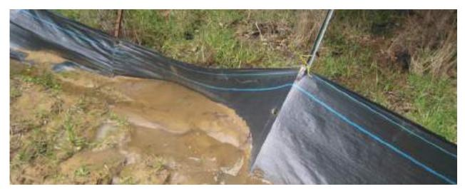
This silt fence is not properly installed and sized causing failure.
