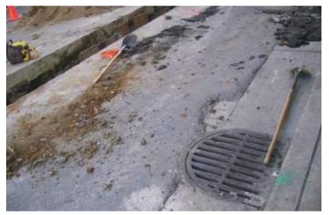
This drain inlet is completely unprotected while construction activities are conducted close by, allowing pollutants to enter the storm drain.
