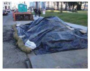
Asphalt debris is escaping from this poorly installed stockpile. Asphalt can release pollutants like hydrocarbons when not properly contained.
