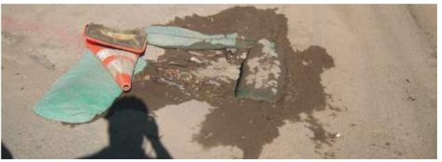
Inspect and maintain all BMP's to ensure that they perform well, and do not fail like this gravel bag berm.
