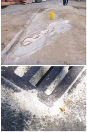
Runoff containing concrete admixtures from unprotected construction activities have made their way to a drainage inlet.
