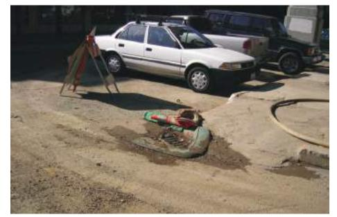
The BMP at this drain inlet needs replacement and ongoing maintenance. Sediment, debris and other pollutants can easily enter the storm drain system.
