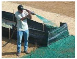
A hydraulic mulch with binder is applied to a disturbed soil area.
