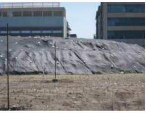
A properly protected stockpile with a plastic cover anchored down by gravel bags.
