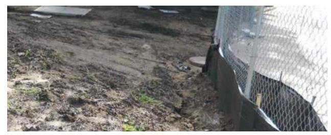
Silt fence is attached to construction fencing to prevent sediment from leaving the site.
