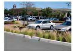
Figure 1-1. Bioretention facilities infiltrate most runoff (above) and can be an attractive landscape amenity (below).
